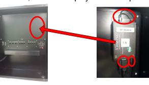
Connect wireless display cable to connector marked inside control box, connect power to UPS, and route antenna cable through hole in the bottom of the control box.
