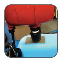
Thread the HydroTronic Control Unit into the fitting on top of the tank. Ensure that the unit is threaded tightly onto the tank. Do not overtighten--.
