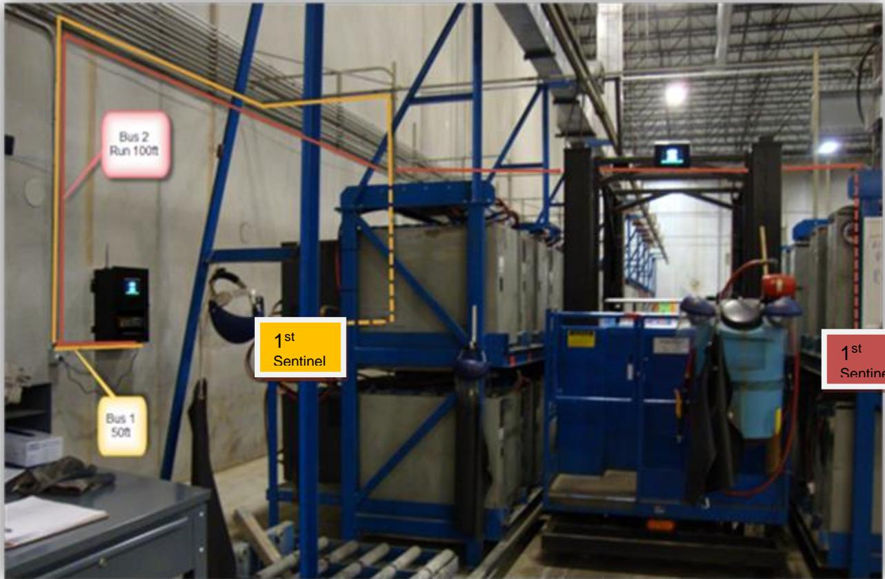
Two examples of Bus cabling are shown in the picture above:
