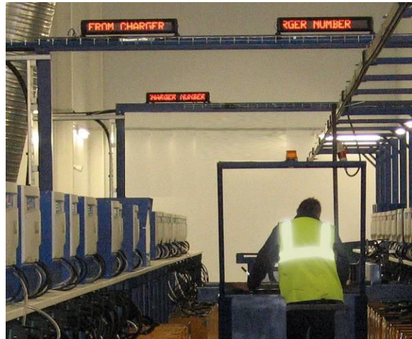
Displays mounted next to each pool of batteries (Method 2)
