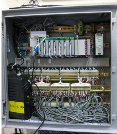
Legacy Control Box, 3 Series PLC Controlled
